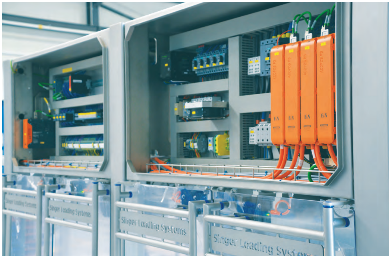
Compact components such as the ACOPOS P3 servo drive give designers more freedom when laying out machines and their control cabinets.
