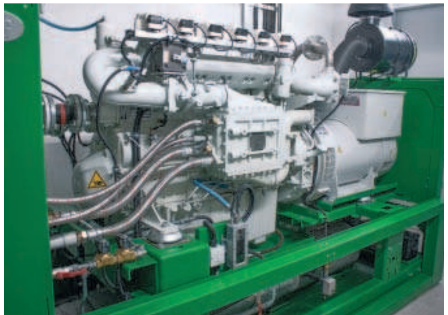
At the heart of the new energy supply system designed and implemented by aeteba is a combined heat and power unit with electrical and thermal capacities of 200 and 256 kilowatts, respectively. Power and waste heat are used primarily to generate energy for refrigeration.
